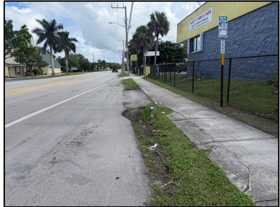
Northbound S.R. 15/E Main Street before the installation of a bus pad. (Pre-Construction)
