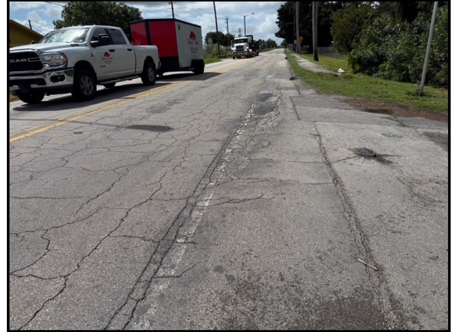
S.R. 15/E Main Street in Canal Point, facing south (Pre-Construction)
