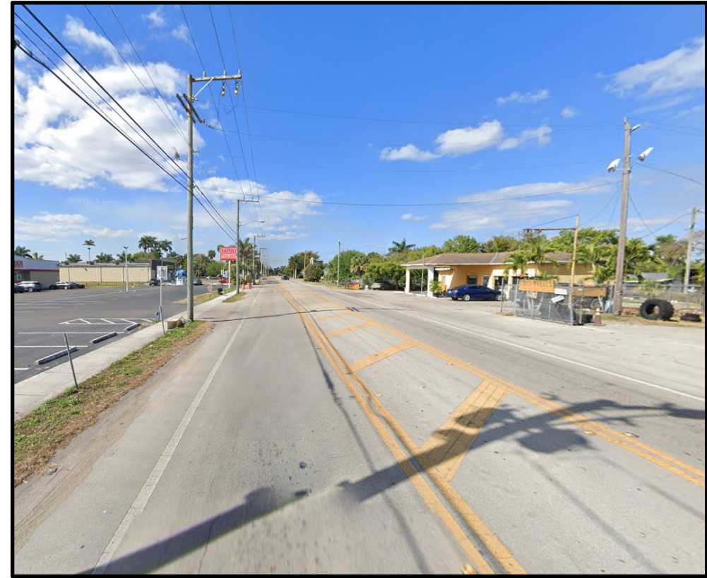
S.R. 15/E Main Street looking south (Pre-Construction)
